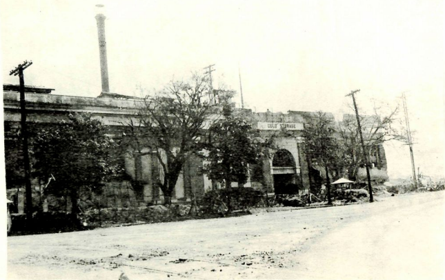
Ice Plant Building Annex 7
