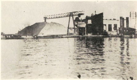
119. Manila Electric Steam Plant. 1939.
