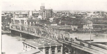
48. Sta. Cruz Bridge over Pasig R., Manila. River spans total about 315 ft. long by 40 ft. wide. Looking N.E. Pre-war.
