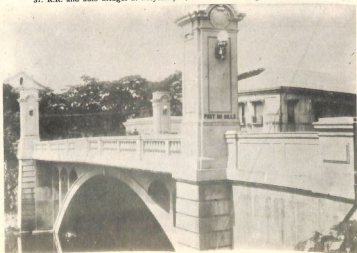
58. Reinforced concrete single arch bridge on Route 3D near San Fernando, Pampanga. Looking north. Pre-war.
