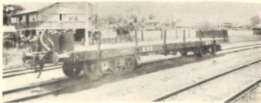
102. Steel bottom Flat Car, 30 tons, Manila R.R. Co.
