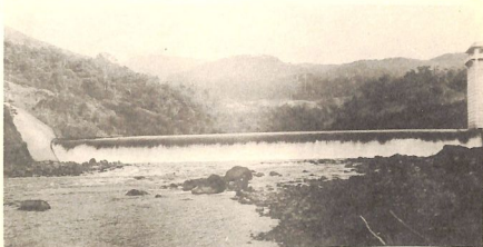
122. Ipo Dam on Angat River, 1939.
