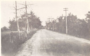
52. Route 3E near Fort Stotsenburg, Pampanga. Two-lane, all weather, black top. Mar., 1944.
