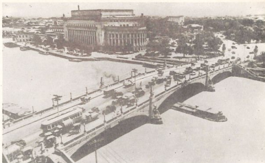
47. Jones Bridge over Pasig R., Manila. River spans total about 325 ft. by 54 ft. wide. Looking east. Pre-war.
