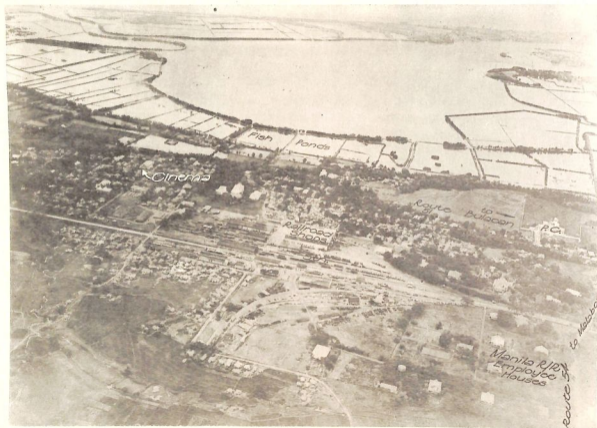
110. Railroad Shops, Caloocan, Manila.
