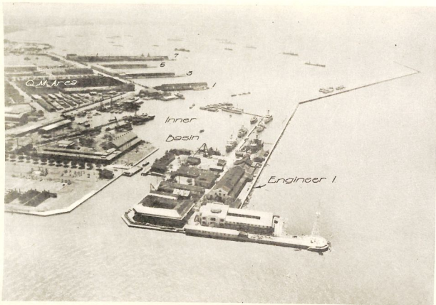
86. Engineer Island and Inner Basin—Manila.
