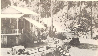
80. Route 7B between Olongapo (Zambales) and Dinalupihan (Bataan). One-lane, all-weather, gravel surface. 1934.
