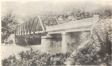
60. Combination steel truss and concrete slab bridge on Route 5E, Digidig, Nueva Ecija. Pre-war.
