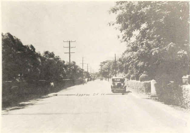
43. Route 1A between Pasay and Paranaque, near Manila. Two-lane, all weather blacktop. 1934.
