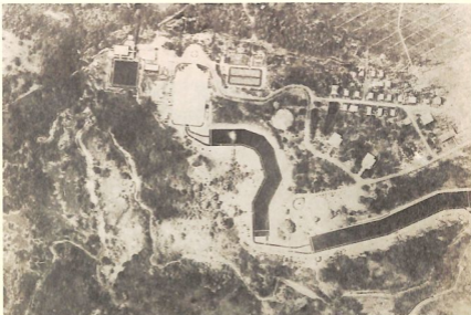
124. Balara Filters—Manila Water Supply. 1940.
