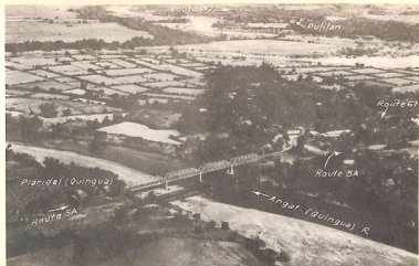
56. R.R. and auto bridges at Plaridel, Bulacan. Looking N.W. Aug., 1938.
