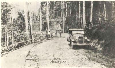
78. Route 7B between Olongapo (Zambales) and Dinalupihan (Bataan) under construction. One-lane, all weather. Pre-war.
