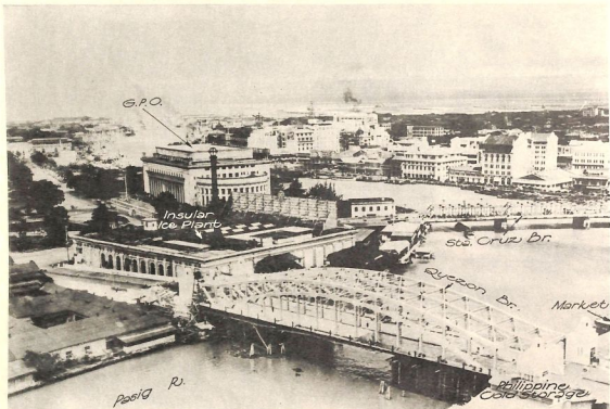
50. Quezon Bridge over Pasig R., Manila. River span, one 336 ft. arch, 65 ft. wide. Looking west. Aug., 1940.
