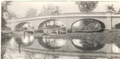
83. Concrete multiple arch bridge on Route 21B at Darangan, Rizal. Looking west. 1927.
