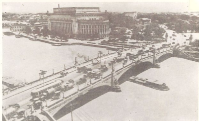
47. Jones Bridge over Pasig R., Manila. River spans total about 325 ft. by 54 ft. wide. Looking east. Pre-war.
