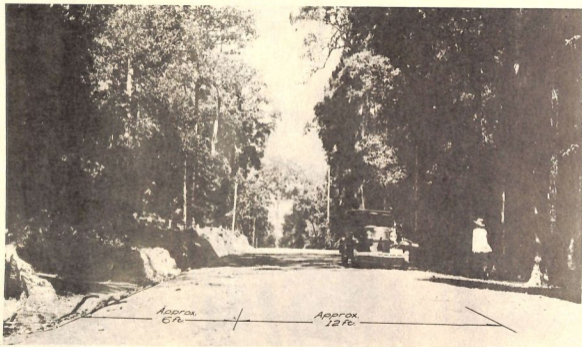
79. Route 7B between Olongapo (Zambales) and Dinalupihan (Bataan). One-lane all-weather, gravel surface. 1934.
