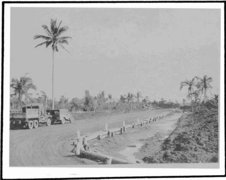
heavy construction equipment made the final road an excellent one.
