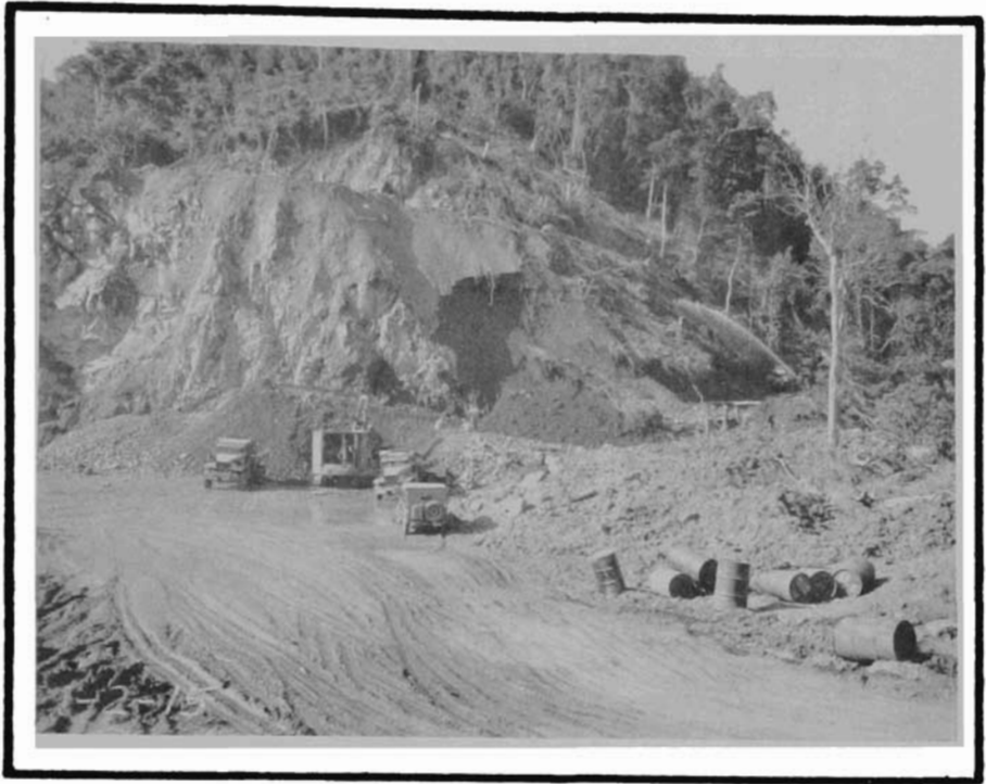
Supplying materials for the roads and bridges were quarries at SALUG and other points on LEYTE,
