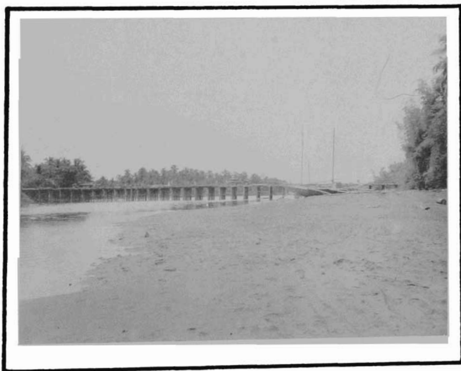
this on the DULAG-ABUYOG road in addition to many others withstood the elements.
