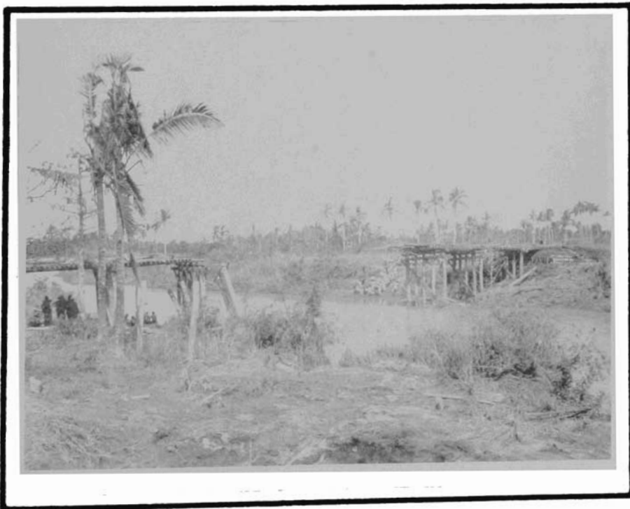
heavy rains in January 1945, which also destroyed the BITO RIVER beach pile bridge.
