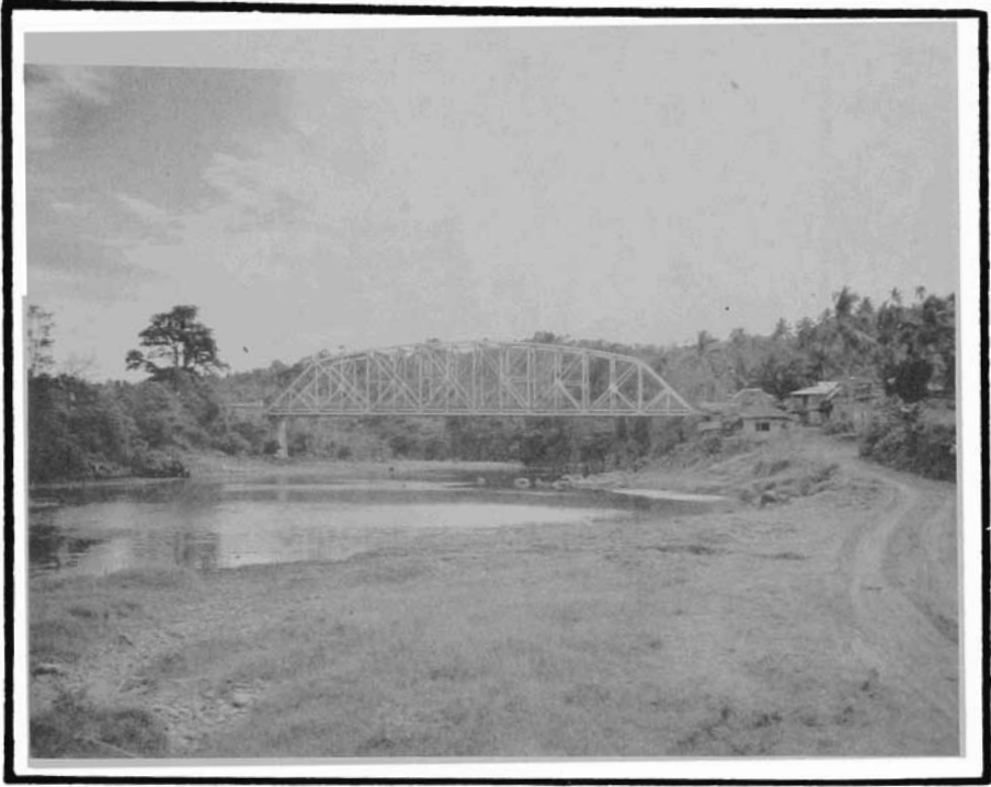
An undestroyed steel bridge between ABUYOG and BAYBAY and
