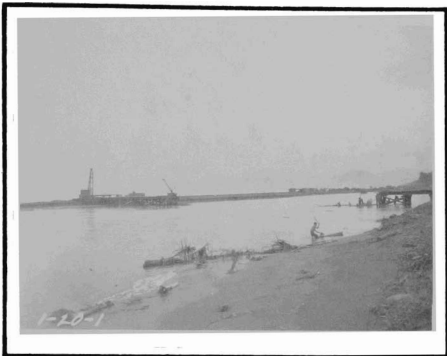
The pile bridge constructed over the BINAHAAN RIVER near DAGAMI was washed out by
