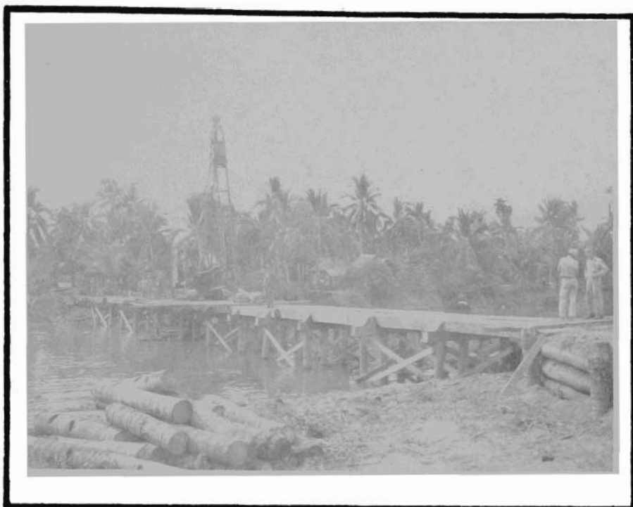
Some pile bridges did not wash out. This one at BAYBAY and
